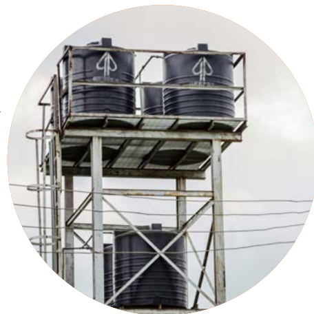
Borehole constructed for 1000 people in Ajoki and Ajamimogha Communities of Edo State
